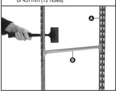
2 Knock the beam **3** with a rubber mallet at both ends to ensure the studs are fully located in the bottom of the keyholes
